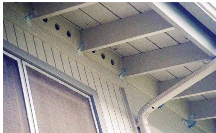
Roof-to-wall hurricane clips can help your roof stay put in a storm.
